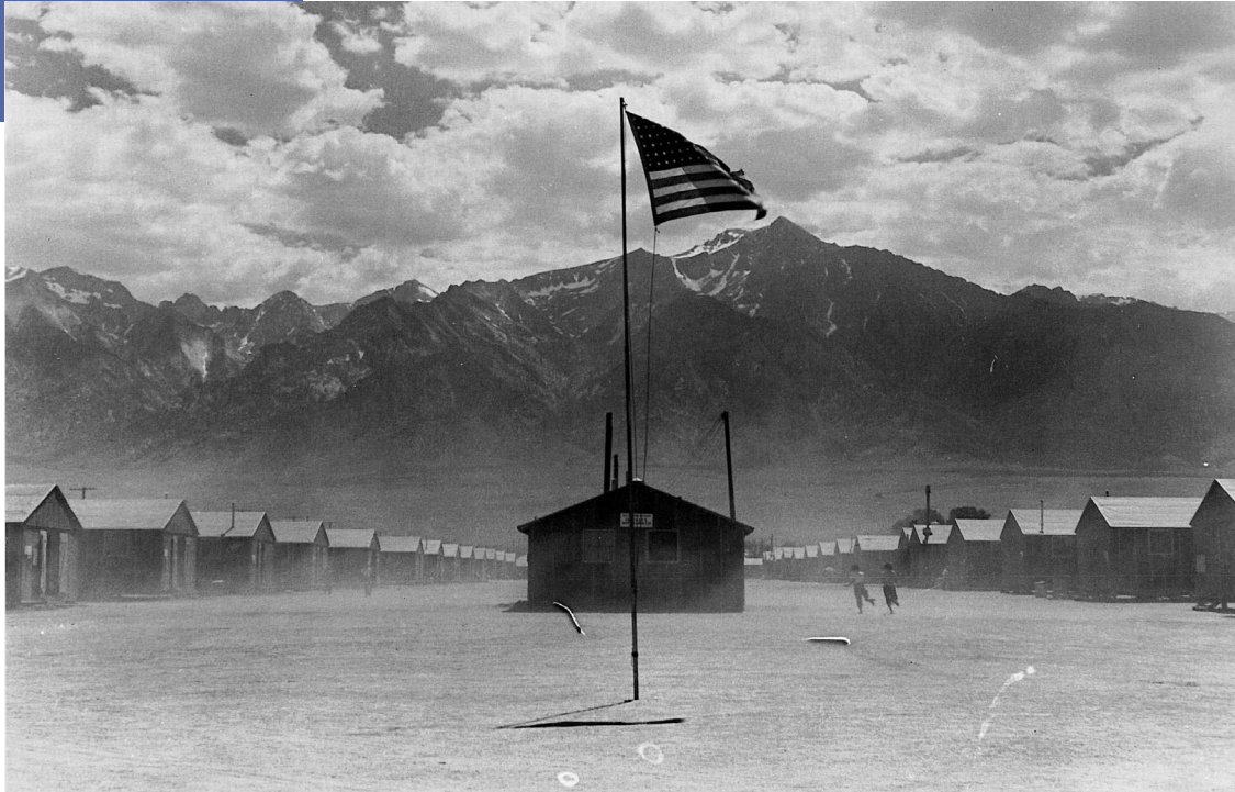
12 DPA Series: RELOCATION OF JAPANESE-AMERICANS — Seventeen prison-type Relocation Centers were built to incarcerate the 110,000 Japanese-Americans. These camps were laid out and constructed on remote Indian reservations, notoriously the most dismal of federally owned property. Operating under the direction of the War Relocation Authority (WRA), each family was assigned a 20 by 25 foot "apartment" in a tarred paper barrack with little furniture and privacy, and no stove or running water. Each 12 barracks, freezing in winter and sweltering in summer, was served by a mess hall, latrines, showers and laundry rooms. The internees maintained all services including the police, fire, and post office departments, and were paid $12 to $19 a month according to their skills (doctors received $19 a month). The 30,000 school children continued their education in poorly equipped classes which, nevertheless, met state standards. The picture shows the Manzanar Relocation Center on a hot and dusty day in July, 1942.
